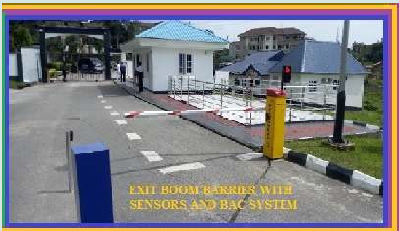
Fig. 2: EXIT BOOM BARRIER WITH SENSORS
