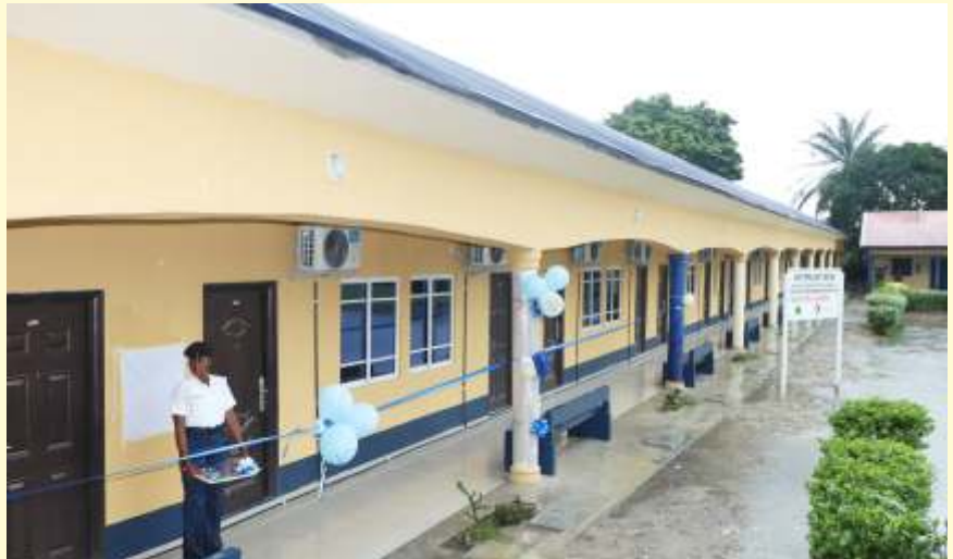
The newly remodelled 20 self contained accommodation for officers
