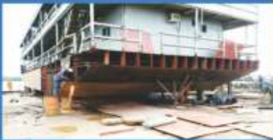
House boat construction and repairs
