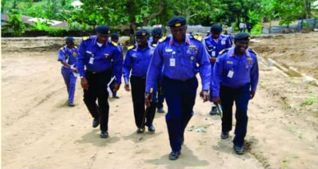
The FOC inspecting the NN Atimbo Barracks perimeter fencing and the road construction
